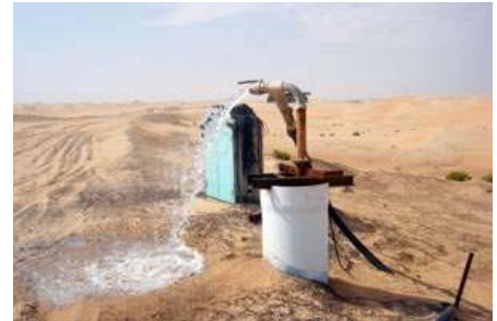
A congested well in the Western Region is cleared using the Airburst developed in the US. Courtesy Impact Porter Novelli
